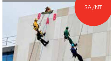
Abseilers dropped down the side of the 10-story building
